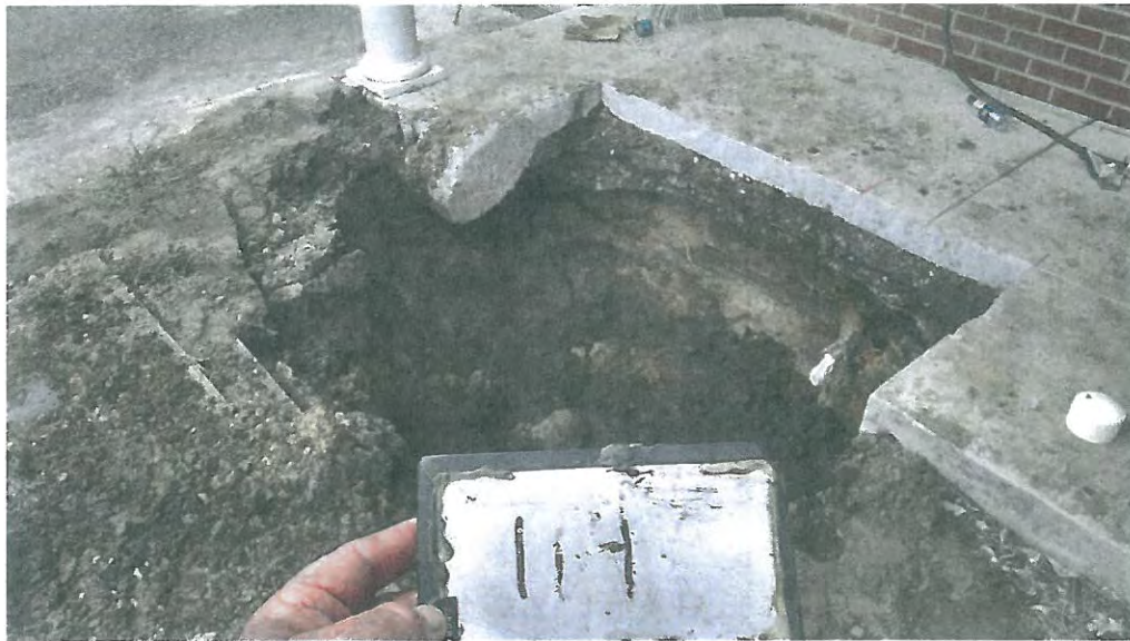
Picture 3: Tank pit.
