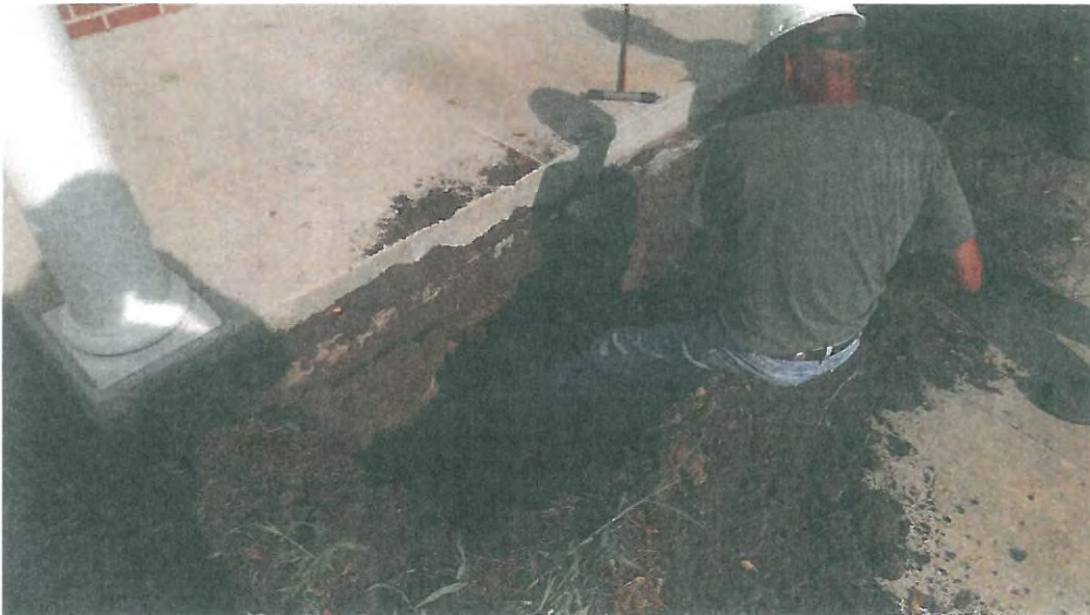
Picture 2: Excavation in progress.
