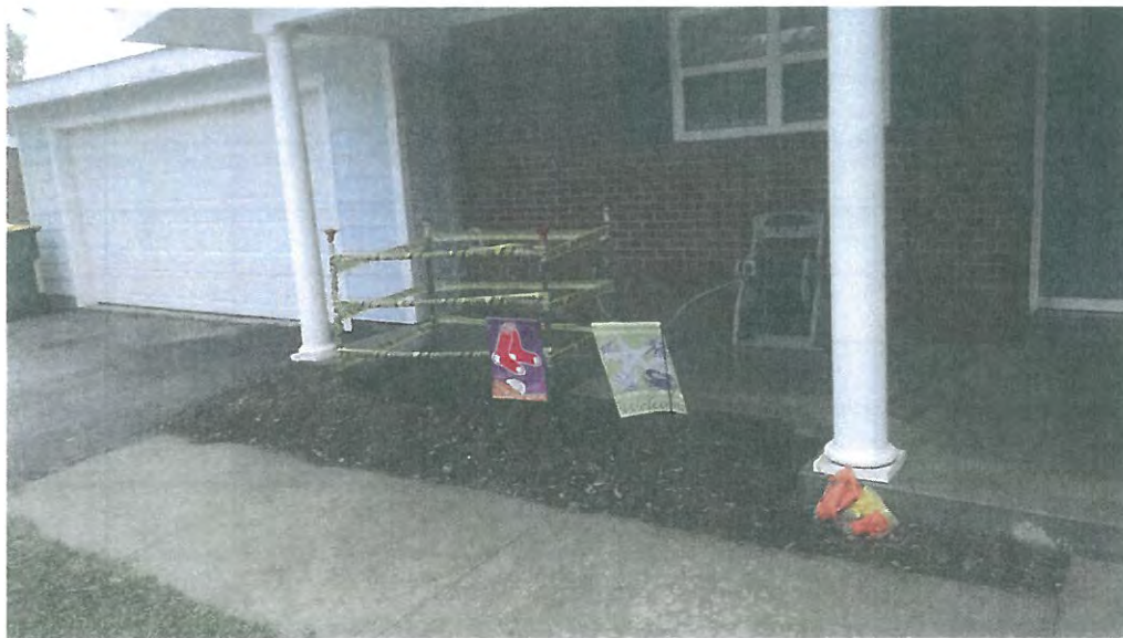
Picture 3: Site after completion of work.
